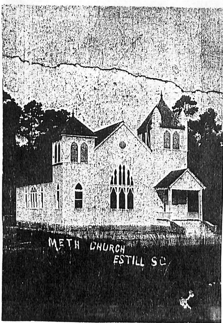
Estill United Methodist Church - General Contractor and one of the founding members, Julian Edgar Rhodes.
